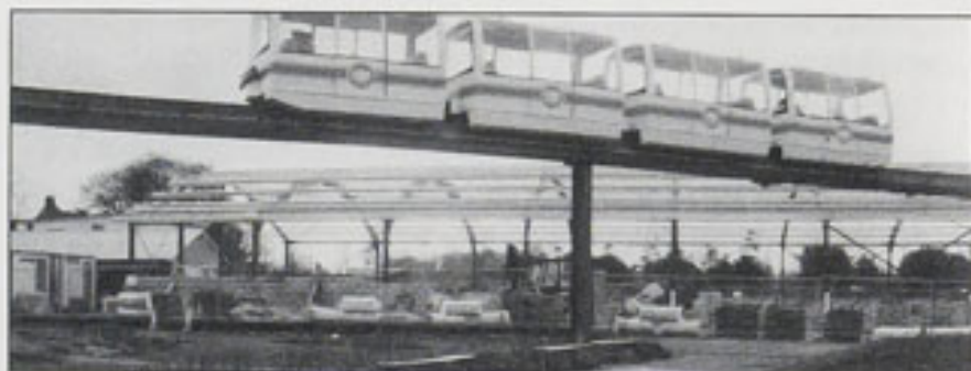
Structural steelwork for Islands in Danger .
