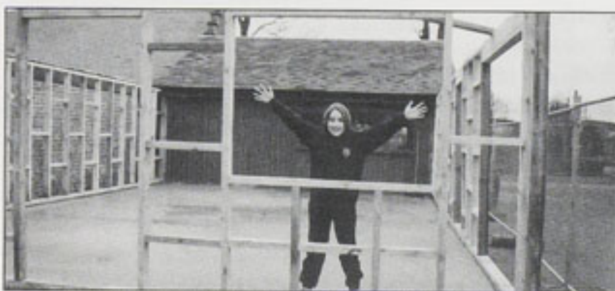
Foundation slab and wooden uprights for the new Wildlife Activity Centre
