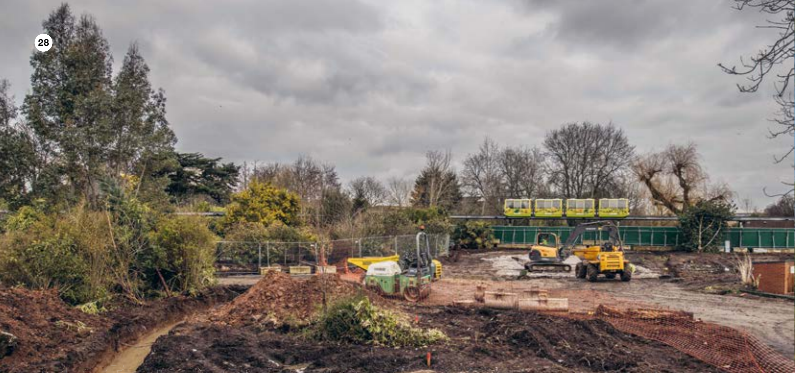
Building works for the lemur walk-through experience
