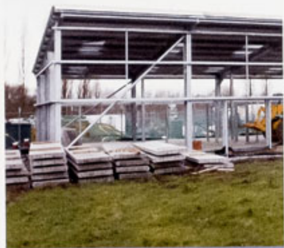
The new Rhino House under construction
