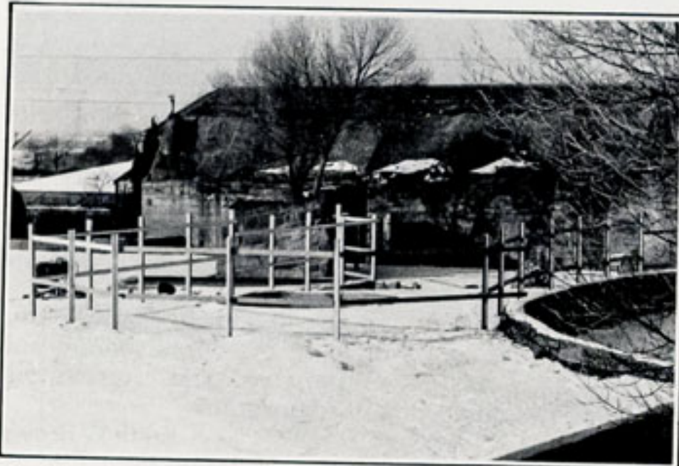
Outside enclosure from top of bridge
