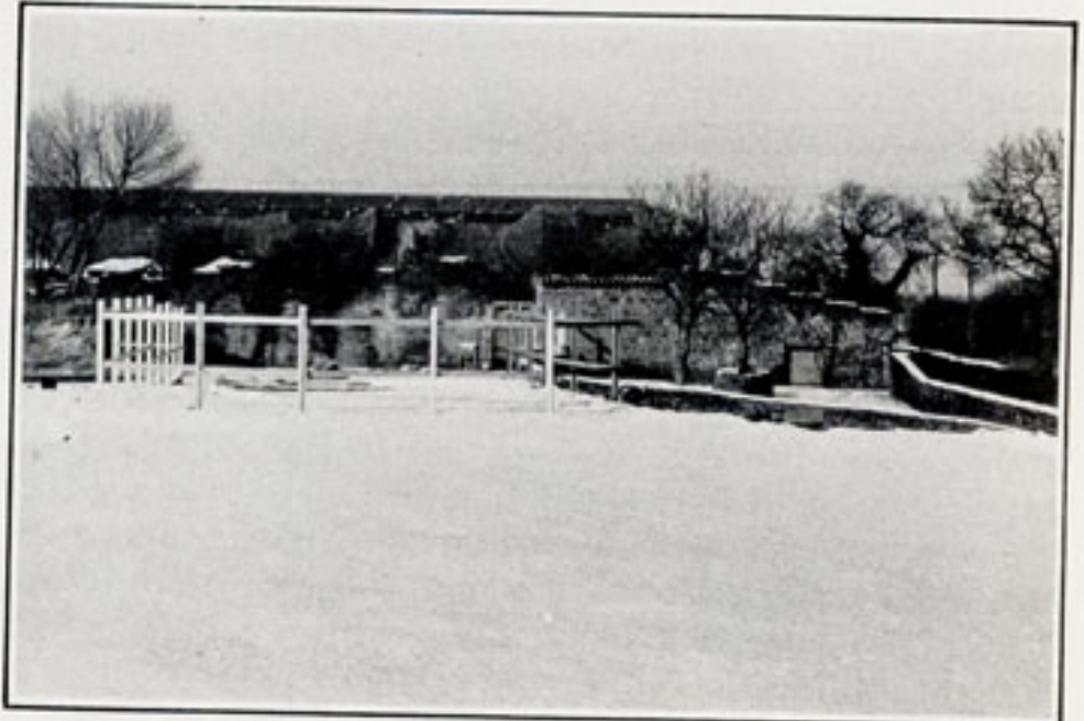
Enclosure from bottom of bridge
