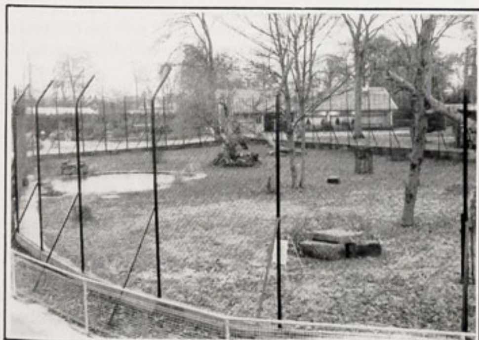
New Tiger enclosure under construction
