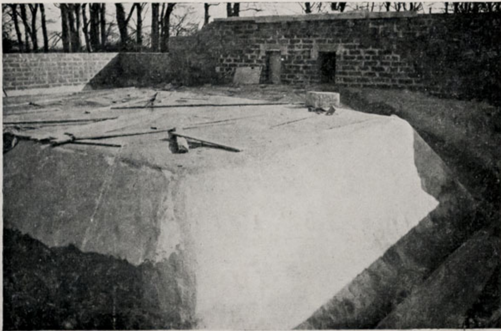
The Brown Bear enclosure under construction.
