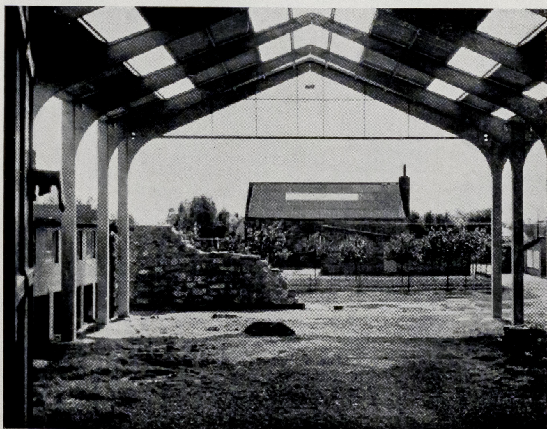
PART OF THE TROPICAL HOUSE NOW UNDER CONSTRUCTION R. T. Bloom
