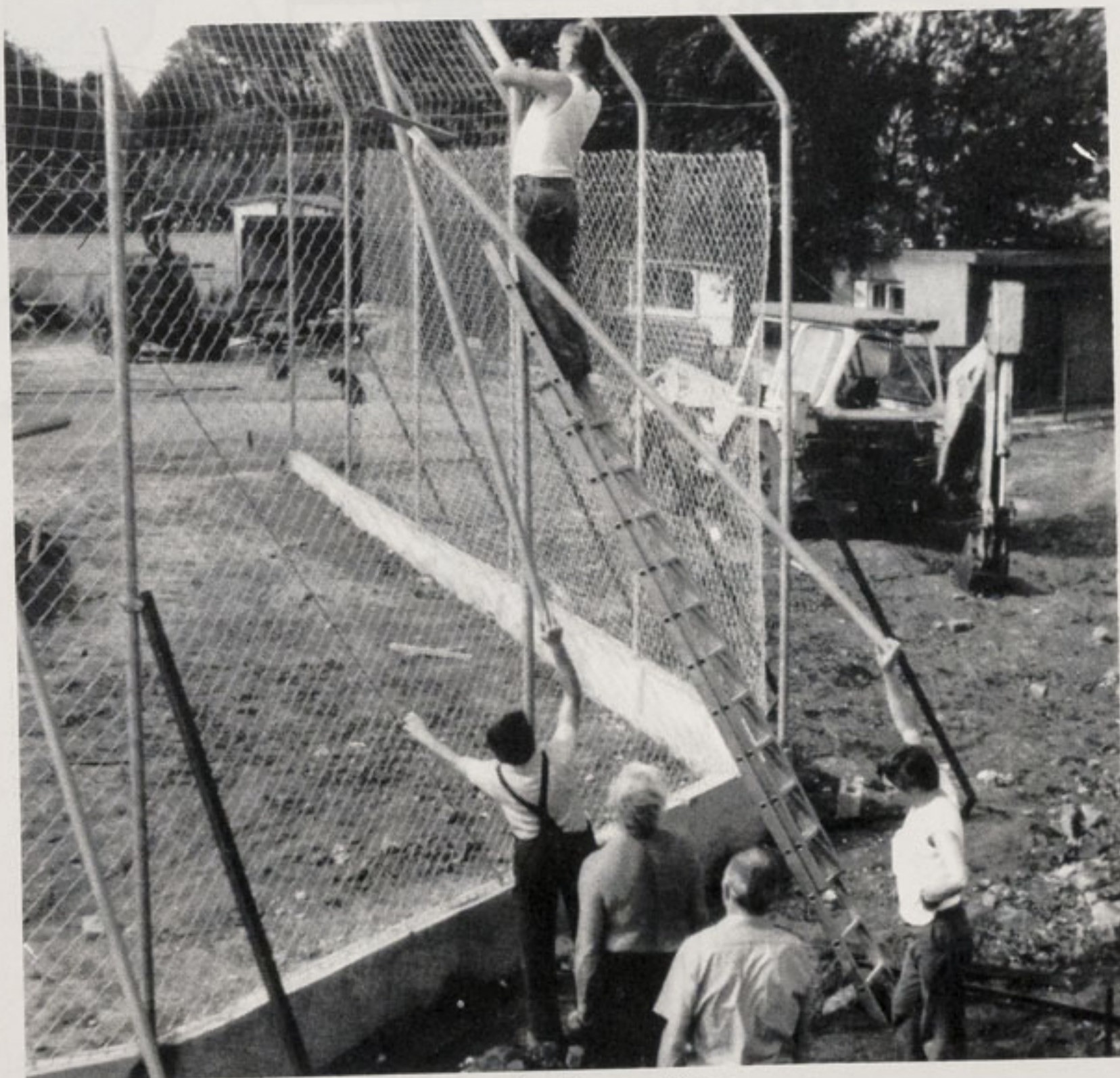
Constructing a tiger-proof fence Courtesy of M. F. Coupe
