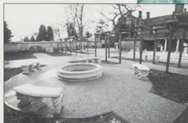
Roman Garden approaching completion
