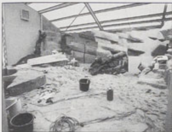
'Rockwork' being built for the Komodo Dragon enclosure
