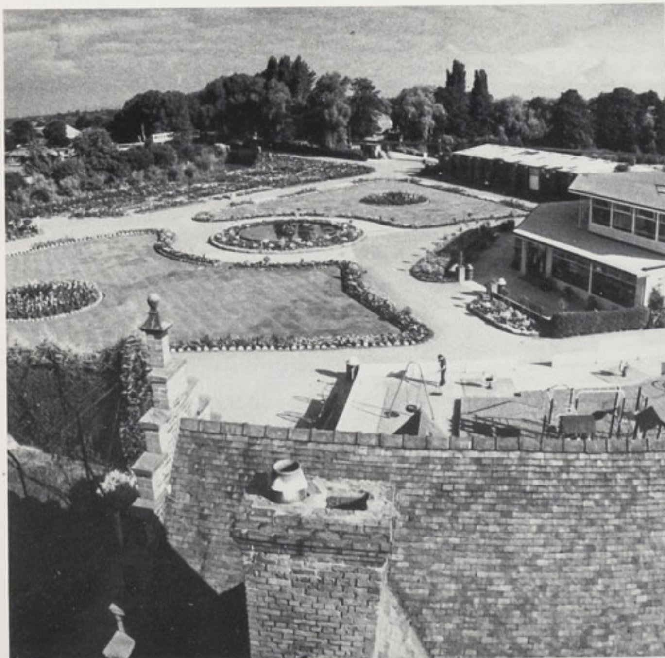
A view from the scaffolding on the Stable Block Spire.
